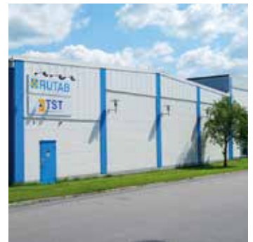
Warehouse - and production facility in Nässjö, Sweden
