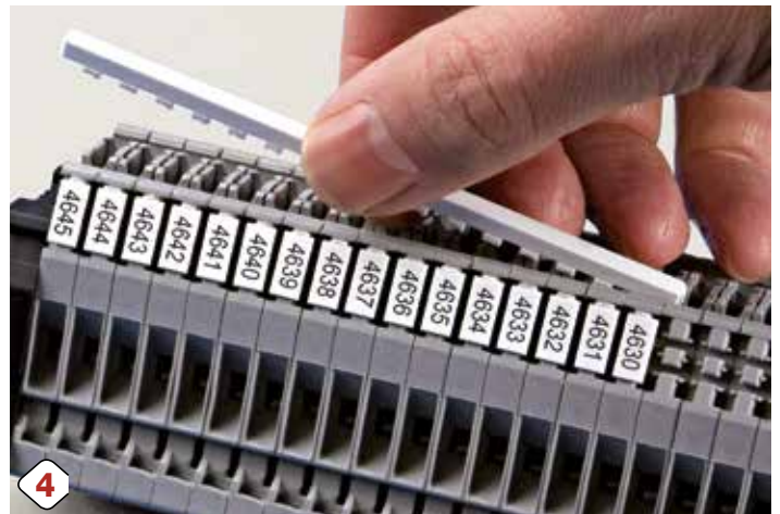
Remove the remaining stem, turning it downwards.
