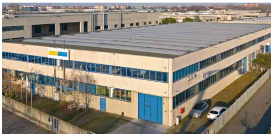
Head office and Logistic Center in Buccinasco, Milan
