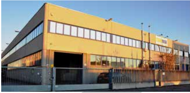
Headquarter and Logistic Center Milan (IT) www.teknomega.it
