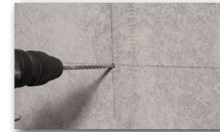
1 Drilled hole Ø 6 mm.
