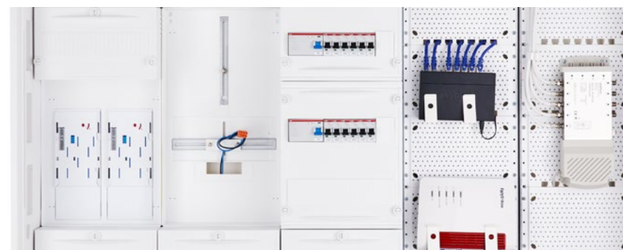
Meter cabinet systems from page 138
