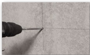
1 Drilled hole Ø 6 mm.
