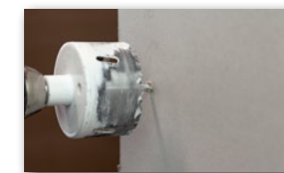
5 Drill into preset hole on opposite side with centering drill of milling crown; counter-sink box hole.
