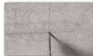
1 Drilled hole Ø 6 mm.
