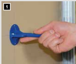
1 Glue the pipe bracket on the back of the first cladding.
