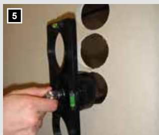
5 Inserting the template.
