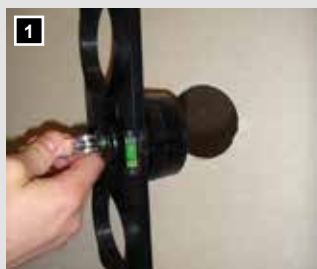
1 Drilling a central hole
