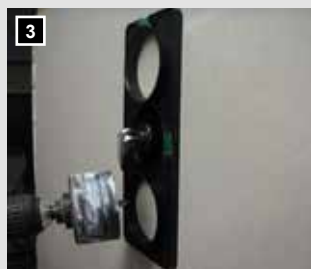
3 Then drill through the existing hole inserts.
