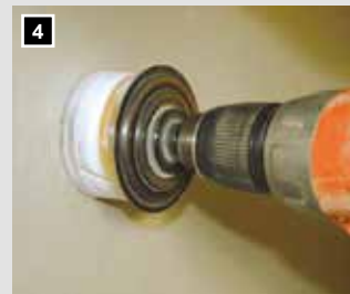
4 You can mill the hole without re-measuring the mounting location.
