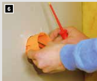
6 Without a long time searching for cables, you can install the cavity wall box.
